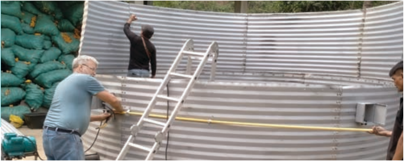
Setting up the dryer bin
