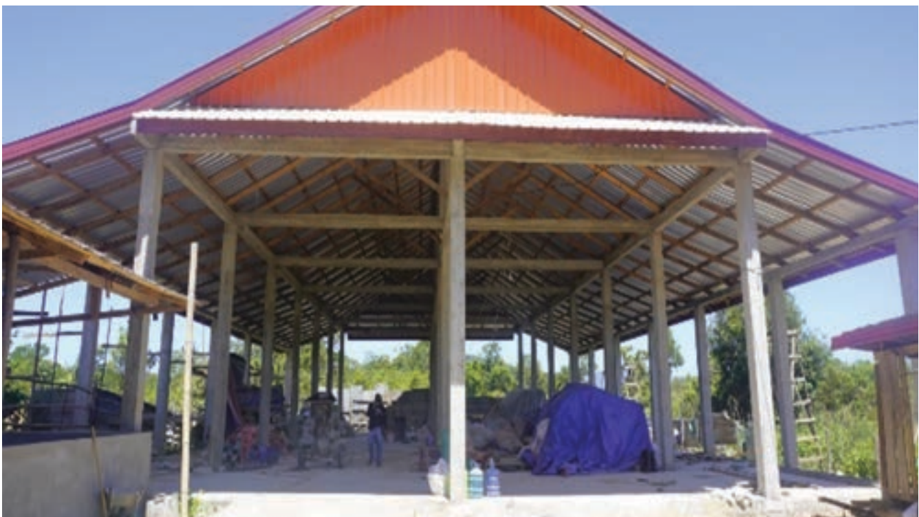
Improved shed ready for harvest: note open sides to promote airflow to prevent mold
