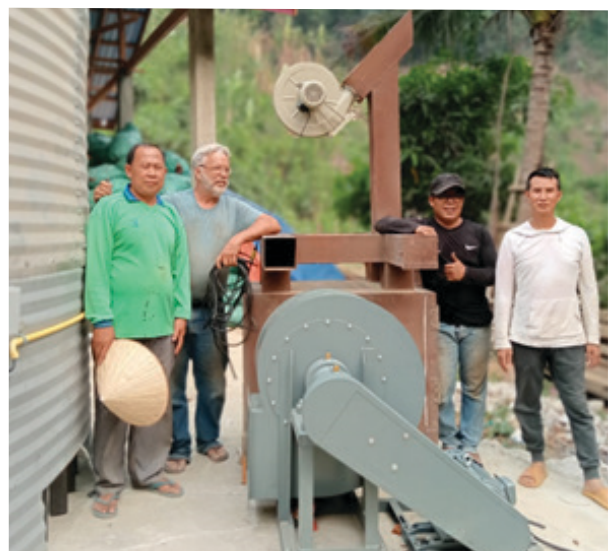
The experts are setting up the fan of the dryer
